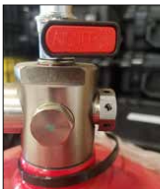
FIGURE 23: Firetrace valve
